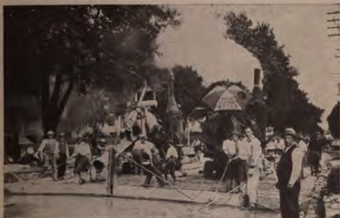
Laying Pavement at Oshkosh, Wis.
